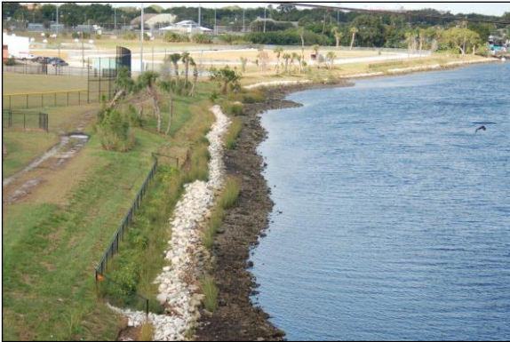
Photo: Stewart Middle School "Living Shoreline" post-restoration: mosaic of estuarine plants, geoweb and rock
