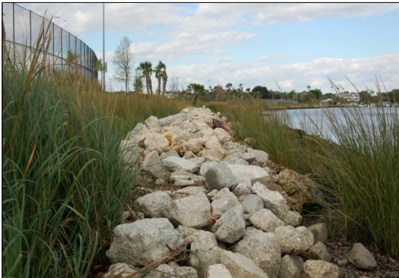
Photo: Stewart Middle School "Living Shoreline" post-restoration: mosaic of estuarine plants, geoweb and rock
